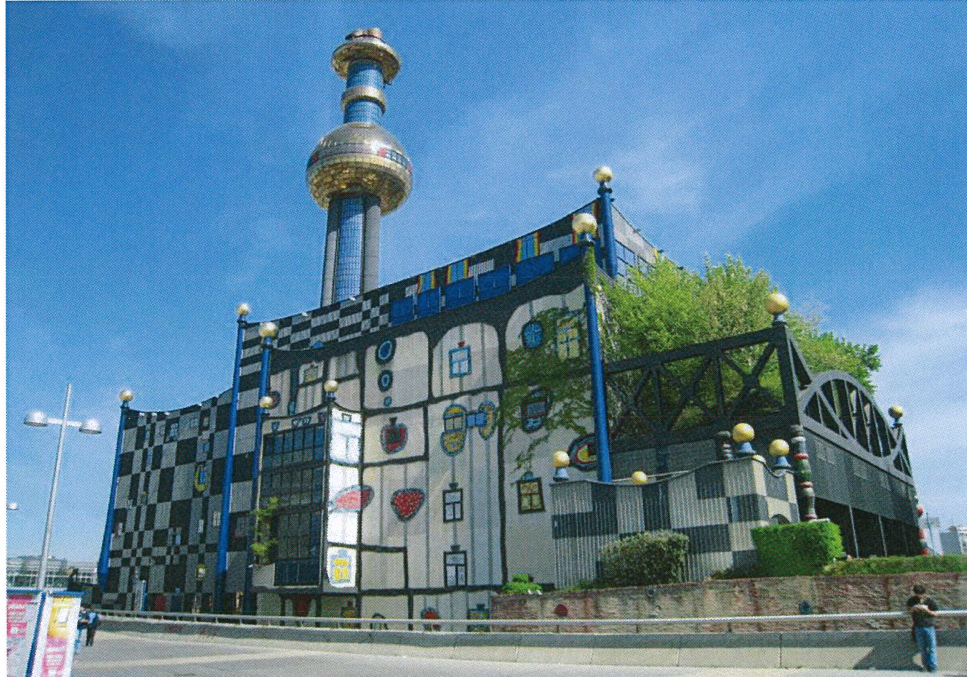
Example 1: Spittelau incineration plant in Vienna, Austria, designed by famous painter and designer Friedensreich Hundertwasser.
