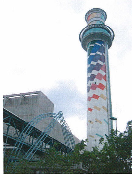
Example 4: Incinerator in Beitou, Taipei, with a revolving restaurant at the top of the chimney.
